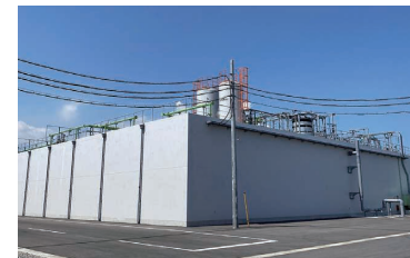
Wastewater treatment facility, Fujibo Ehime's Oita Plant
